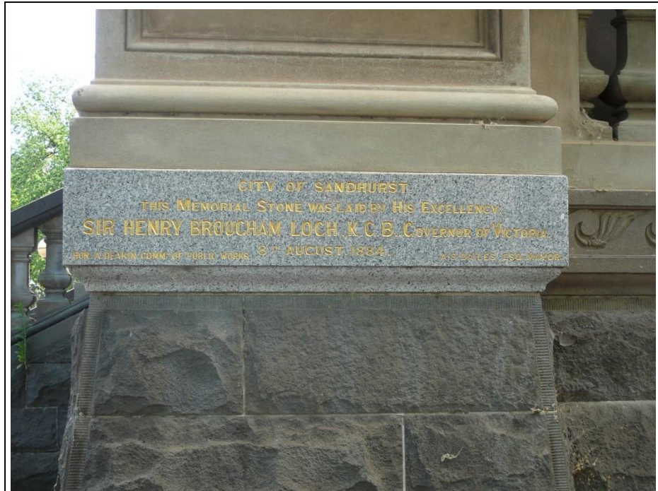
Figure 7. Harcourt granite foundation stone of the Bendigo Public Buildings, unveiled in August 1884 [Photo: Susan Walter, 2022]
