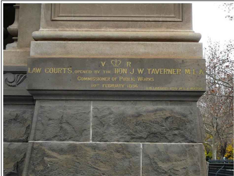
Figure 9. Bendigo Court House “Opening Stone” from 10 February 1896, with the memorial carved into Malmsbury bluestone. [Photo: Susan Walter, 2022]
